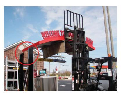
**STEP 2**: The steel posts (or post) need to be anchored in place prior to lifting canopy on top. Make sure the 45 degree angle is facing the back (see red circle in picture)
