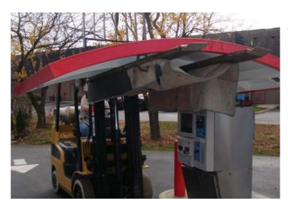
**STEP 3**: Lift canopy up and line it up with canopy steel post (or posts).
