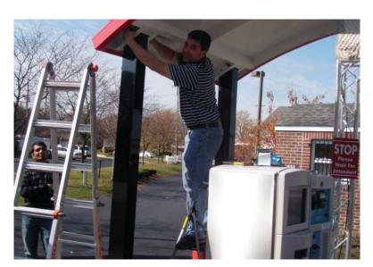
**STEP 4**: Once the post (or posts) are inserted inside the canopy, slide the long bolts in(supplied with the canopy).
