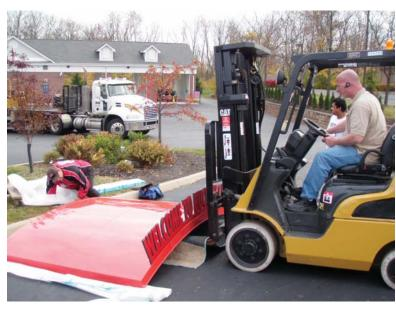
**STEP 1**: Use the foam that is used in shipping the canopy to protect it when its laid on the ground or from fork arms.
