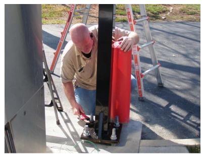
**STEP 6**: You may have to shim it to make the post levelled. Once the post is levelled then tighten all bolts.
